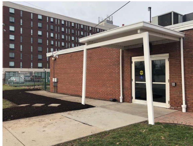
Mary's Home front entrance
